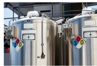
On storage tank
